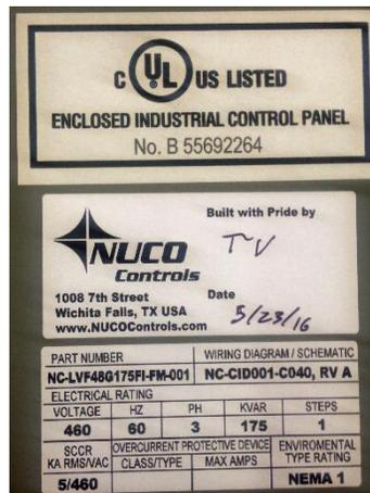
Figure 2: UL certification sticker on top and nameplate on bottom
