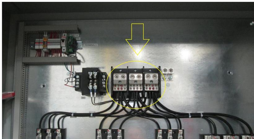
*Figure 6: Capacitor bank power cables connection to distribution block*
